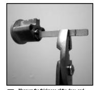
Measure the thickness of the door, and using pliers, break off the 2 connecting screws and the tailpiece on the back of the cylinder to the appropriate length. [see table above, noting whether you are installing a single or a double cylinder lock] (CAUTION: Measure the door and cut the screws and tailpiece carefully. Cutting them too short or allowing them to be too long will result in improper installation/operation of the lock.)
