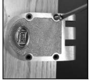
Using the 4-2" mounting screws and a screwdriver, attach the deadbolt to the inside of the door using the 4 small mounting holes drilled earlier.
