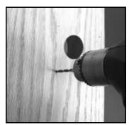
Carefully drill the 4 smaller mounting holes (1/8" drill bit) in the inside of the door to a depth of 3/4". (CAUTION: Use care to limit the depth of the hole to 3/4" to avoid drilling completely through the door.)
