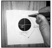
Place the point of the center punch directly on the center of the 4 small mounting holes and the large cylinder hole marked on the installation template and strike with a hammer to transfer the marks onto the surface of the door and the door trim.
