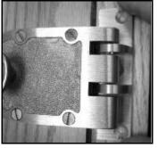
Set the lock strike in place and set the lock in the locked position. Allign the strike on the door jamb with the lock strike centered on the bolt. Make sure there is no interference between the bolt and the strike when operating the lock. Mark the position of the strike, and then unlock the door and open it. Mark the center of the mounting holes for the strike and drill 1/8" holes where marked. It may be necessary to shim the door frame or to mortise out the frame for proper strike alignment.
