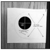
Cut out the appropriate installation template and tape it to the inside of the door at the desired height of the lock. The template will attach to the edge of the door. Take care to position the template properly, aligned to the edge of the door (not the frame) and use a straightedge and level to ensure it is placed perfectly level on the door. (TIP: Use care when taping to ensure that the tape doesn't damage the finish of the door.)
