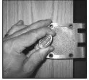
Holding the lock in place, operate the lock from both the inside and outside to ensure smooth operation. If binding is encountered, recheck the thickness of the door and the length of the tailpiece. Re-trim the tailpiece if necessary.
